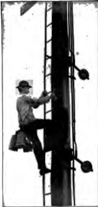
Carrying night lanterns to the top of a railway signal post.
